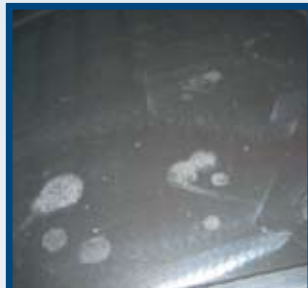
Damage caused by bird/bat stains
